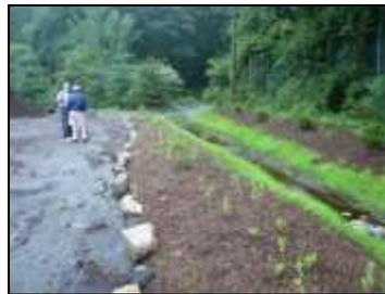
*With the new cascading rain gardens project, run off from the parking lot is filtered slowly through a planted swale and rip rap, filtering the stormwater before it flows into the brook.*
