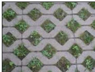
*Turfstone pavers replace the dirt emergency driveway at the rear of the DPW building, slowing the stormwater runoff into the Troy Brook*
