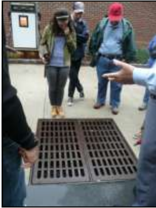
It's not just a grate in the driveway—participants look into the oil water separator at the filling station at the Parsippany-Troy Hills Police Department on Route 46, close to Troy Brook, left.
