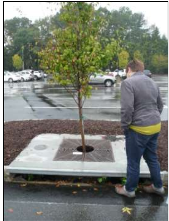
Tree boxes were installed in the parking lot to capture and filter stormwater runoff from this urban parking lot, right. To learn more about tree boxes, visit our website.
